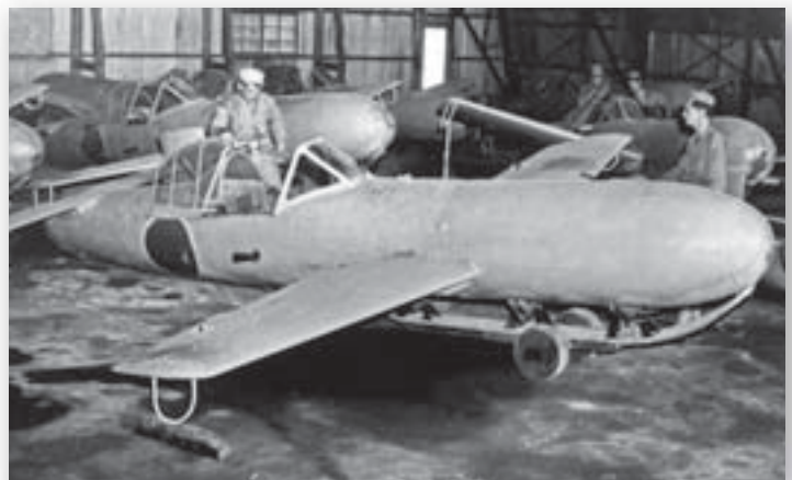
The Ohka K1 was the basic training version of the Ohka and was fitted with a skid under the nose for the return landing. This hanger at Yokosuka is filled with the trainers. (NARA)
