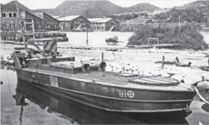
The Type 5 was a detachment leader boat and was larger than the Type 1. It could be fitted with a 13mm machine gun in front of the cabin, but that is absent on this boat, which had been disarmed prior to the US occupation. This boat was part of the Kawatana Assault Group in Ogushi harbor. (NARA)
